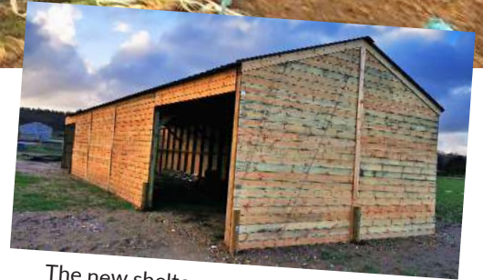
The new shelter nears completion...
